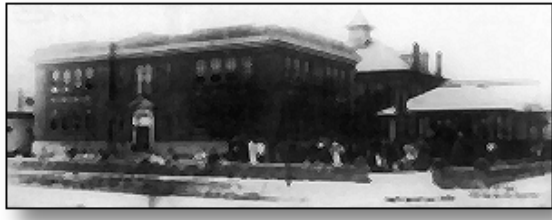
Two Story Hyde Park School Building (Gorrie Elementary)
